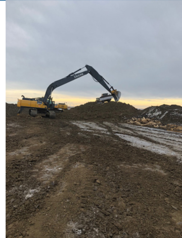
8. Backfill - Km 164+244 – Jan 18, 2018
