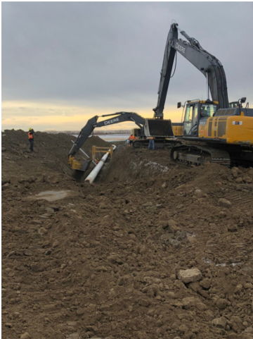
9. Backfill shading mainline - km 162+260 – Jan 18, 2018
