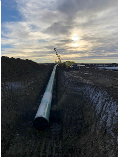
13. Lowering in – Km 166+650 – Jan 19, 2018
