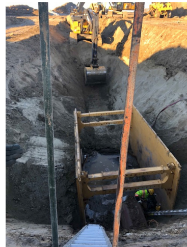
16. Excavator dig – km 159+428 – Jan 20, 2018
