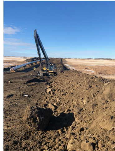
10. Long stick excavator clearing wetland - Km 165+190 – Jan 19, 2018
