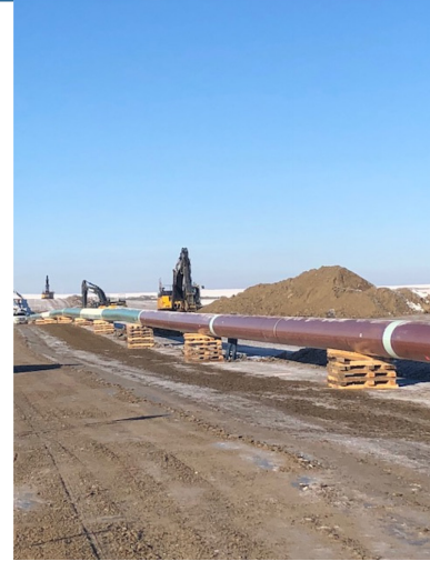
20. Excavators - km170+300 – Jan 21, 2018
