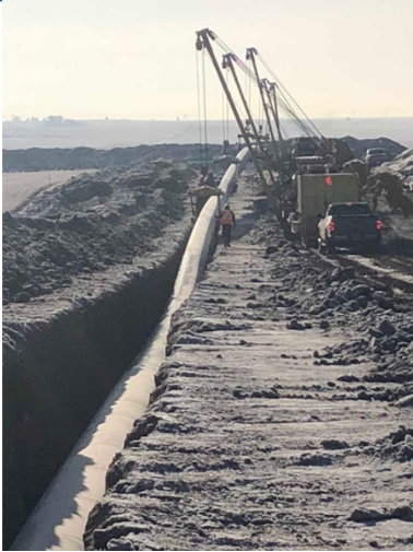
19. Side booms lowering in- km169+200 – Jan 21, 2018
