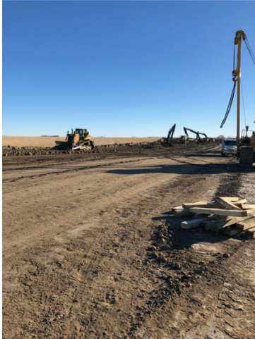
3. Backfill Crew - 164km+050 – Jan 16, 2018
