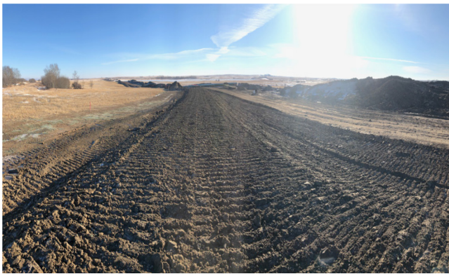
15. Tie-in backfill - km 164+325 – Jan 20, 2018
