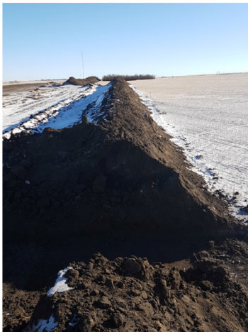
5. Access route (wildlife and run-off) – Km 161+350 – Jan 16, 2018
