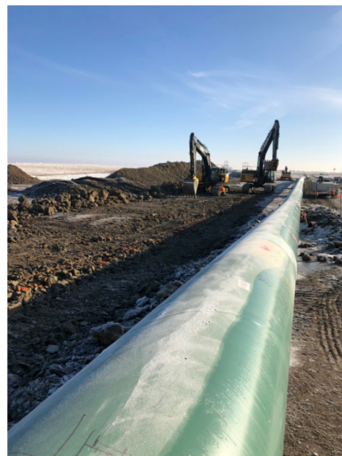
18. Pre-ripped ditch line - km170+200 – Jan 21, 2018
